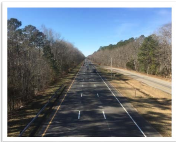
Existing facility looking westbound from weigh station
