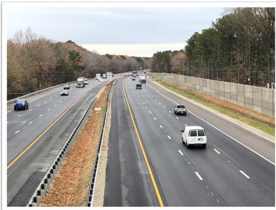
Project Site (Looking West from Denbigh Blvd.)
