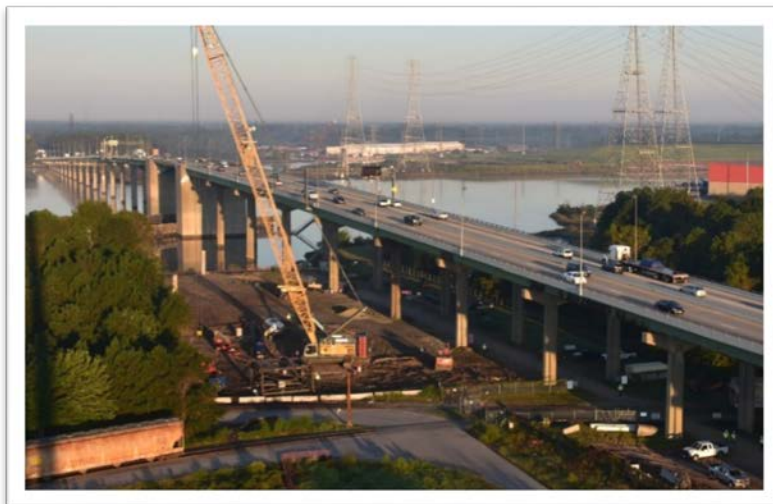
Pile Driving Operations for East Approach Spans of New High Rise Bridge
