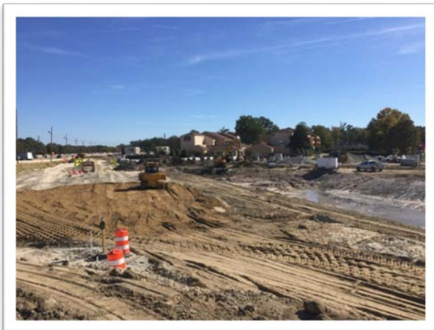
Ground and Drainage Improvements I-264 E (Exit 15 B)
