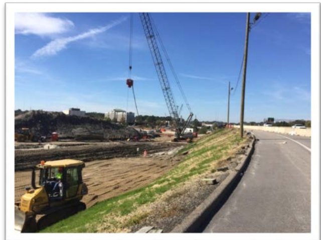
I-264 E Bridge B-601 over Newtown Road (looking west)
