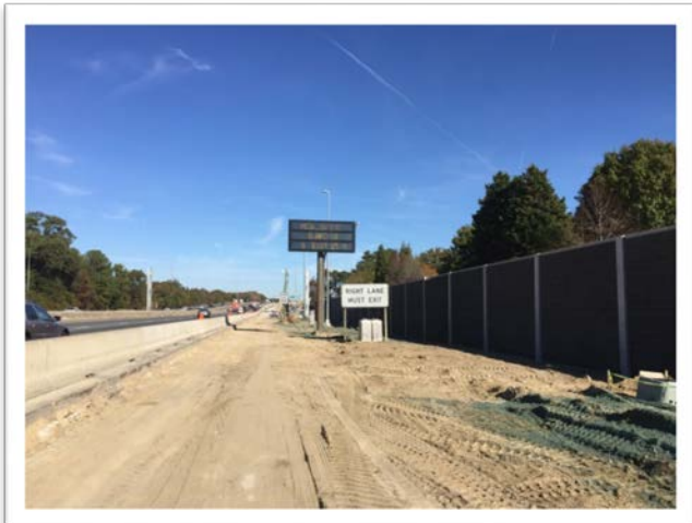
Widening I-64 W and Sound Barrier 2 (Sentara)
