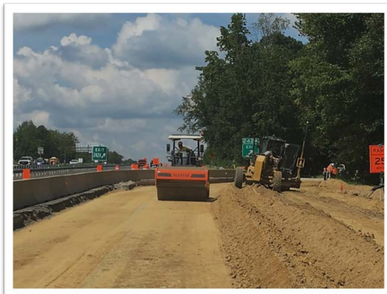
I-64 westbound grading operation at the Exit 242A
