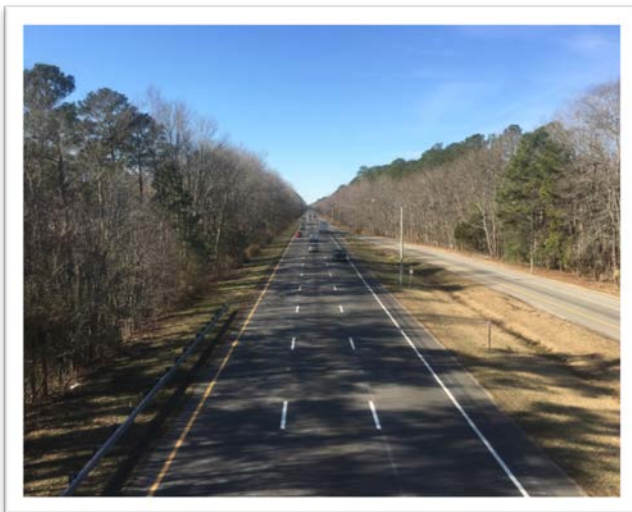
Existing facility looking westbound from weigh station
