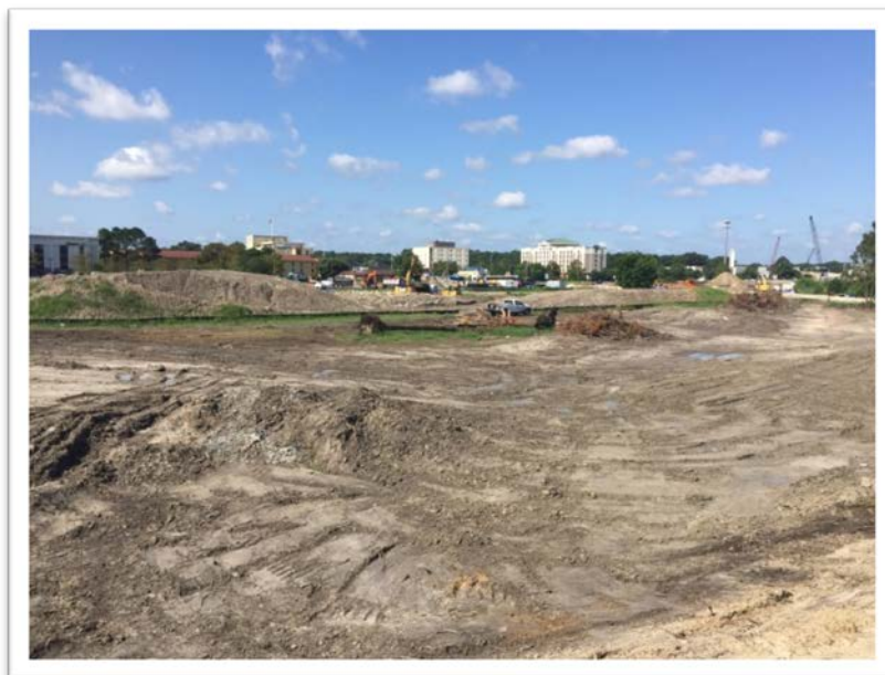
Exit 15 B, I-264 EB; Ground Improvement and Sediment Pond Construction
