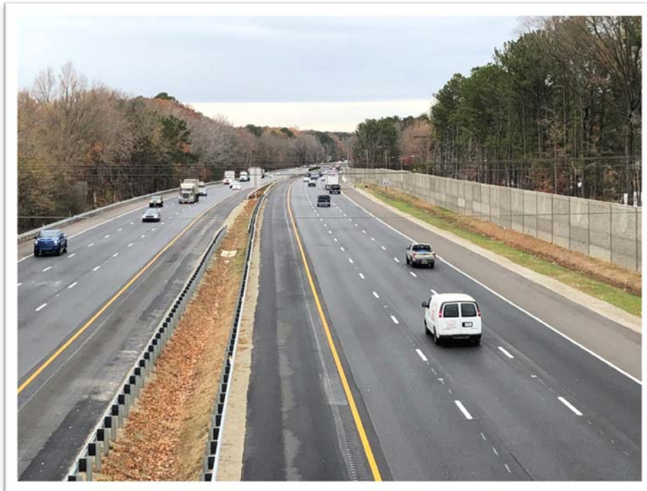
Project Site (Looking West from Denbigh Blvd.)
