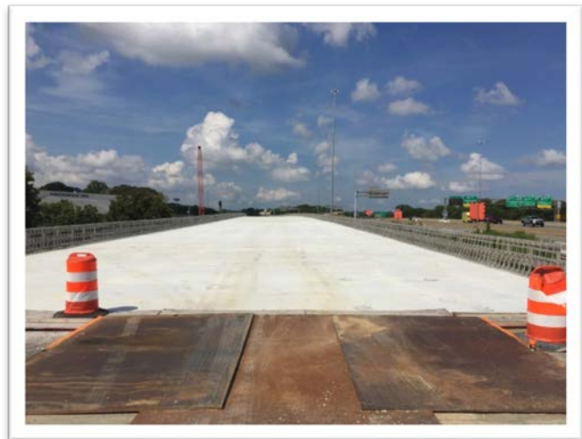
Completed bridge deck B-605 looking west
