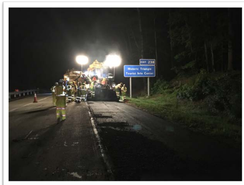
I-64 westbound outside shoulder strengthening operation
