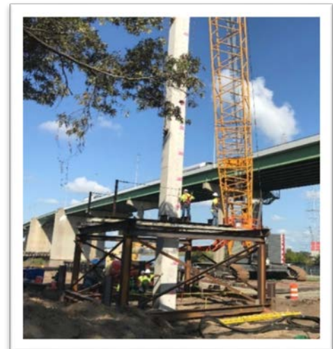
Pile Driving Operations for East Approach Spans of New High Rise Bridge
