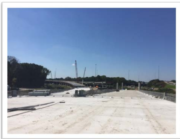
Bridges B-603(l), B-602 (r) and B-605 (foreground)
