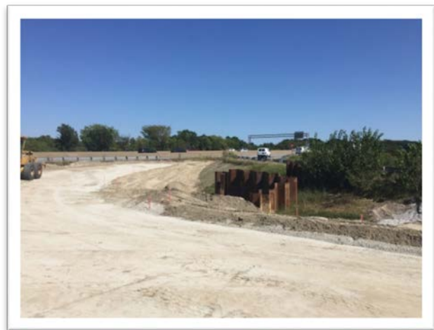
Temporary Loop A; Exit 15A
