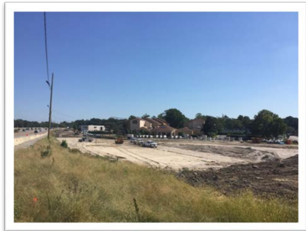
Future Site of Roundabout, I-264 Exit 15A
