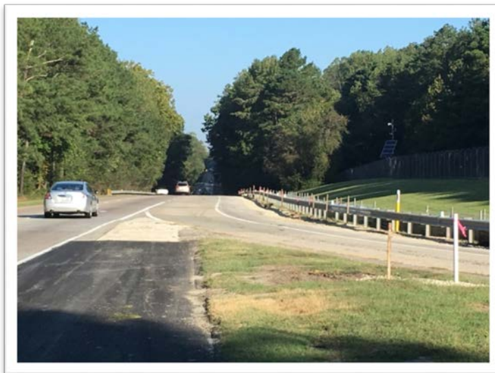
I-64 westbound outside shoulder strengthening and temporary guardrail installation
