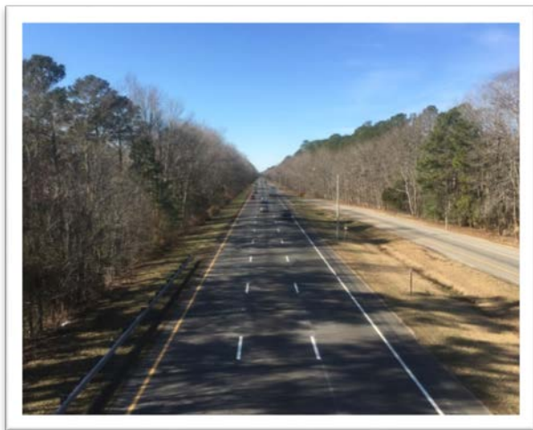
Existing facility looking westbound from weigh station
