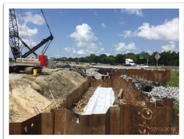
Box Culvert 8-34 Foundation Exit 15A
