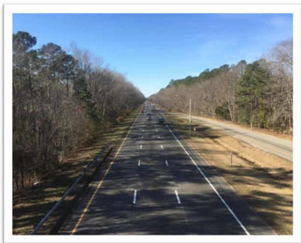
Existing facility looking westbound from weigh station
