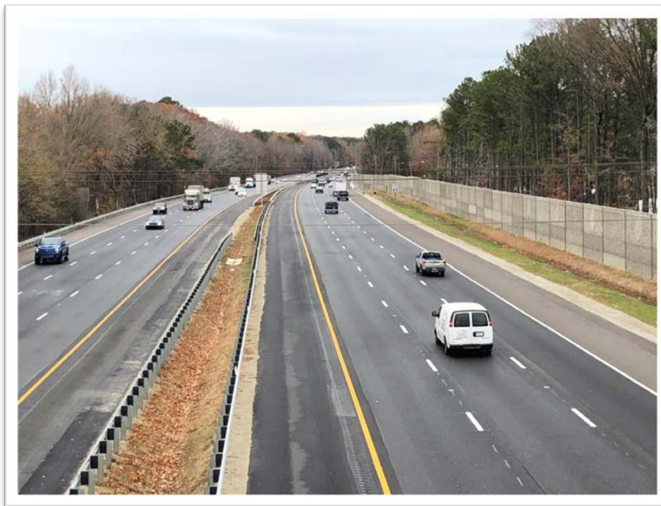
Project Site (Looking West from Denbigh Blvd.)
