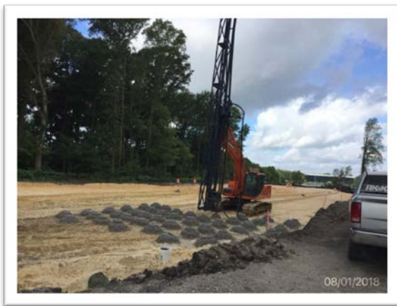
PVD Installation Cleveland Street
