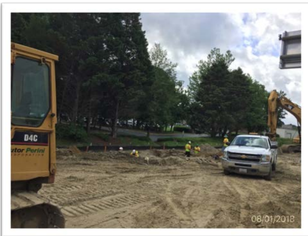
Sound Barrier Footings (Rear of Sentara Nursing Facility)
