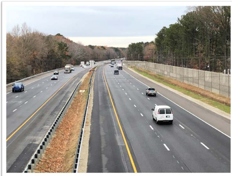
Project Site (Looking West from Denbigh Blvd.)
