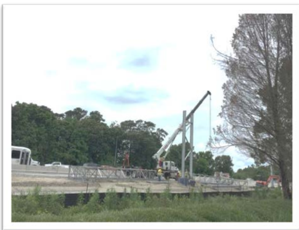
Overhead Sign Structures I 64 W
