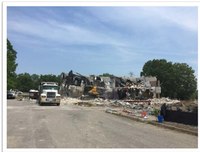
Parcel 016 Demolition - Business Park Drive
