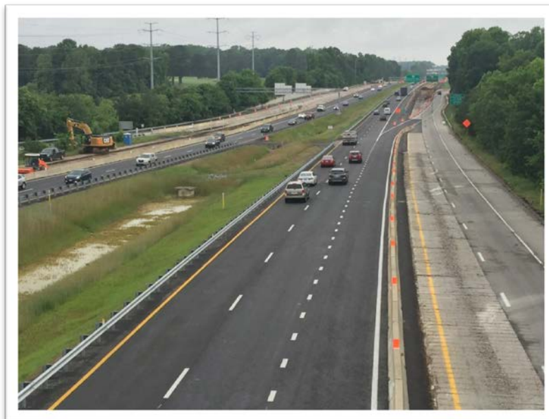
I-64 Westbound Traffic Shift to Phase 2 in Sections A and B
