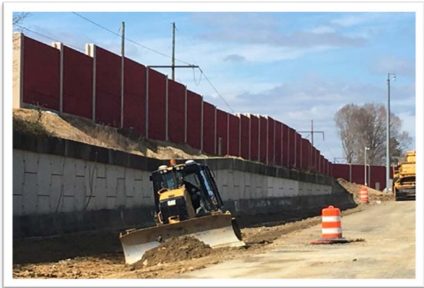
Eastbound I-64 noise wall and ditch grading
