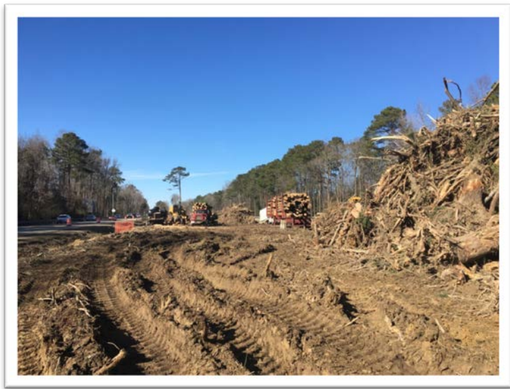
Clearing and grubbing operations in center median of I-64
