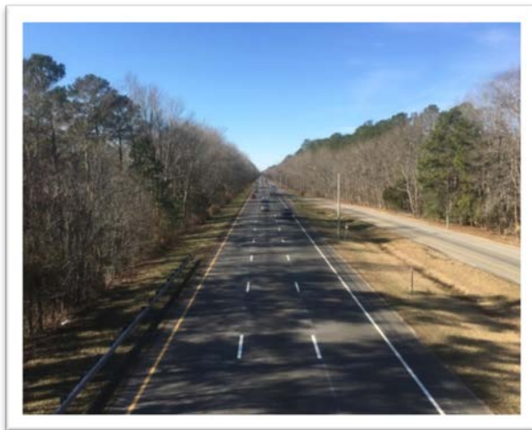
Existing facility looking westbound from weigh station
