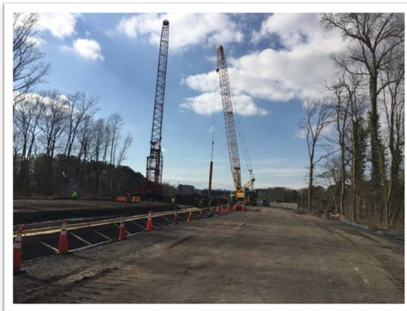
Cleveland Street Approach to B-603; I-264 Flyover
