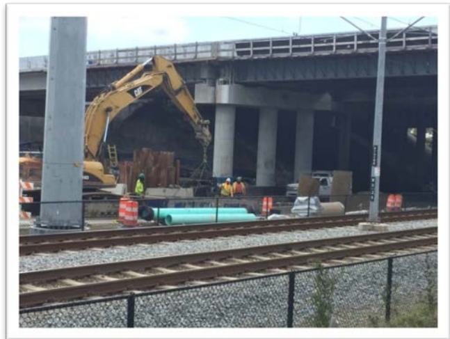
Utility Work Curlew Drive
