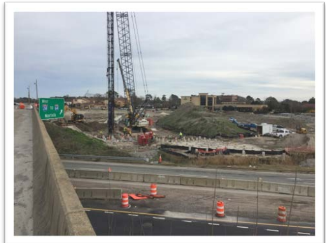
Box Culvert Extension I-264 EB just east of Top Golf
