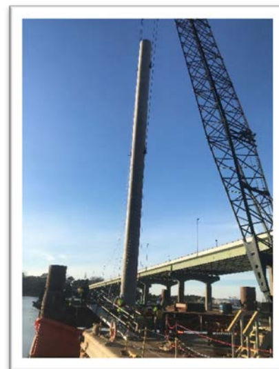
Pile Driving Operations for East Approach Spans of New High Rise Bridge
