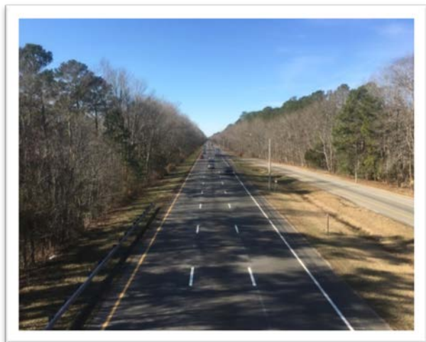
Existing facility looking westbound from weigh station
