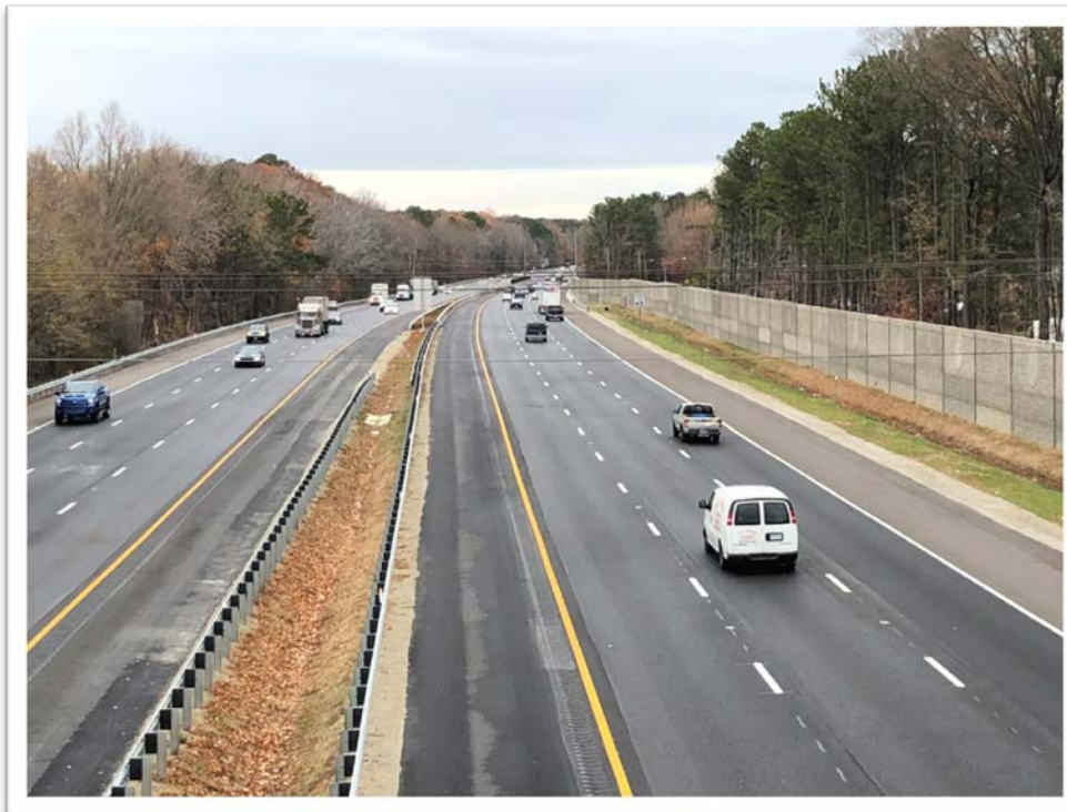
Project Site (Looking West from Denbigh Blvd.)
