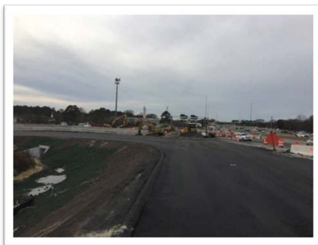
South Newtown Rd Loop to I-264 EB. Culvert 8-34 Inlet (left)
