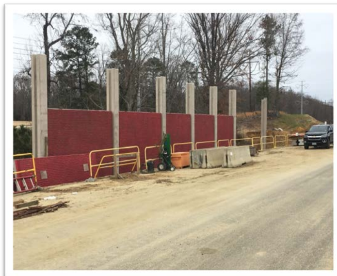
I-64 Noise wall construction
