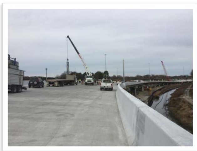
Overhead Signs Bridge B-602
