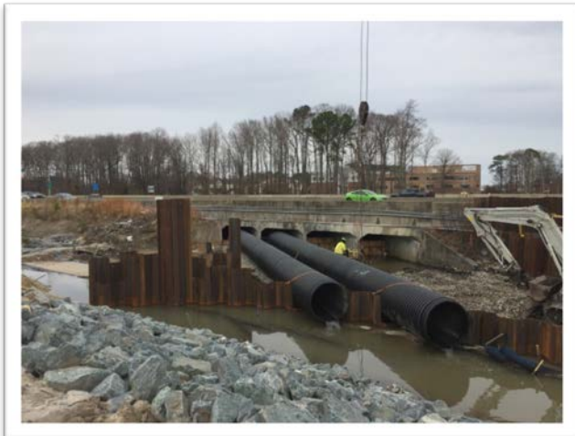
Ground Improvement Piles I-264 Over Newtown Road
