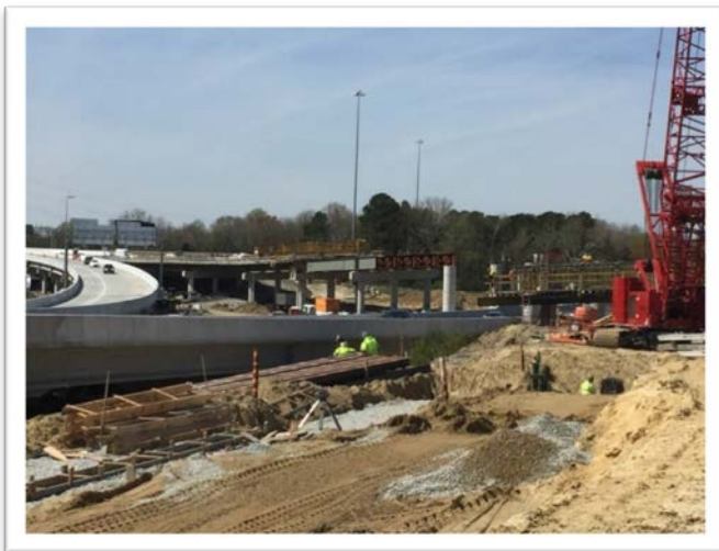
Landing for B-602 Flyover (B-603 left)
