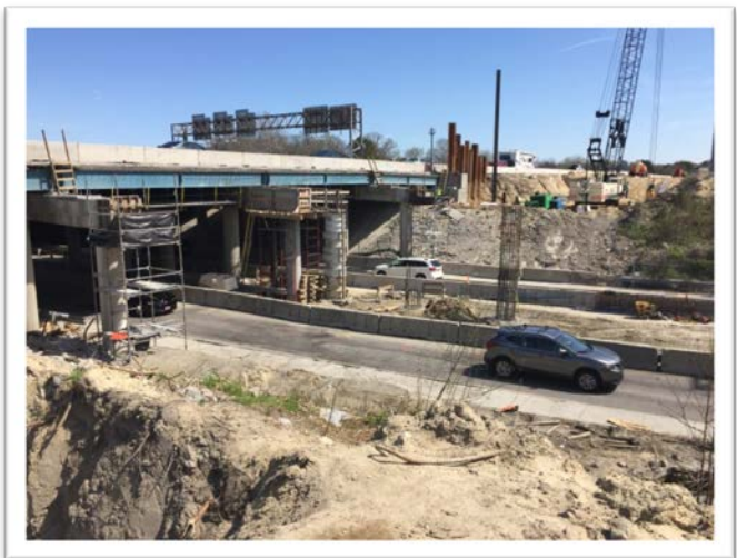
I-264 EB Over Kempsville Road
