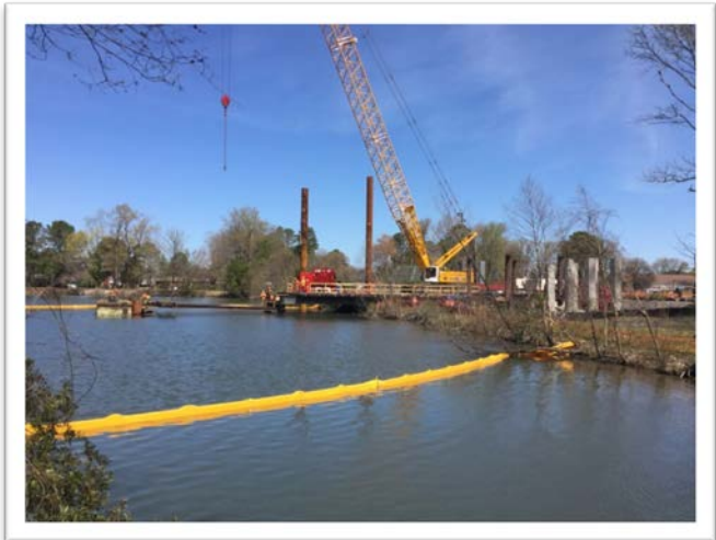
Cleveland Street Work Trestle B-603
