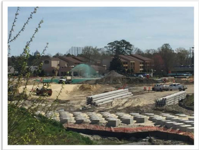
Earthwork and Hydroseeding; Exit 15 I-264 EB
