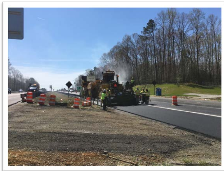
Eastbound I-64 asphalt paving of surface course
