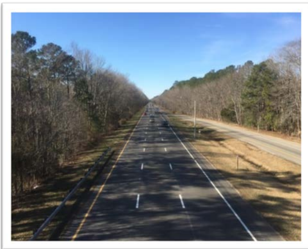
Existing facility looking westbound from weigh station
