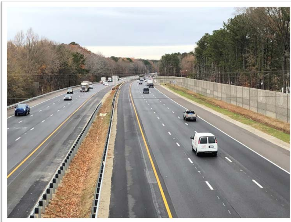
Project Site (Looking West from Denbigh Blvd.)
