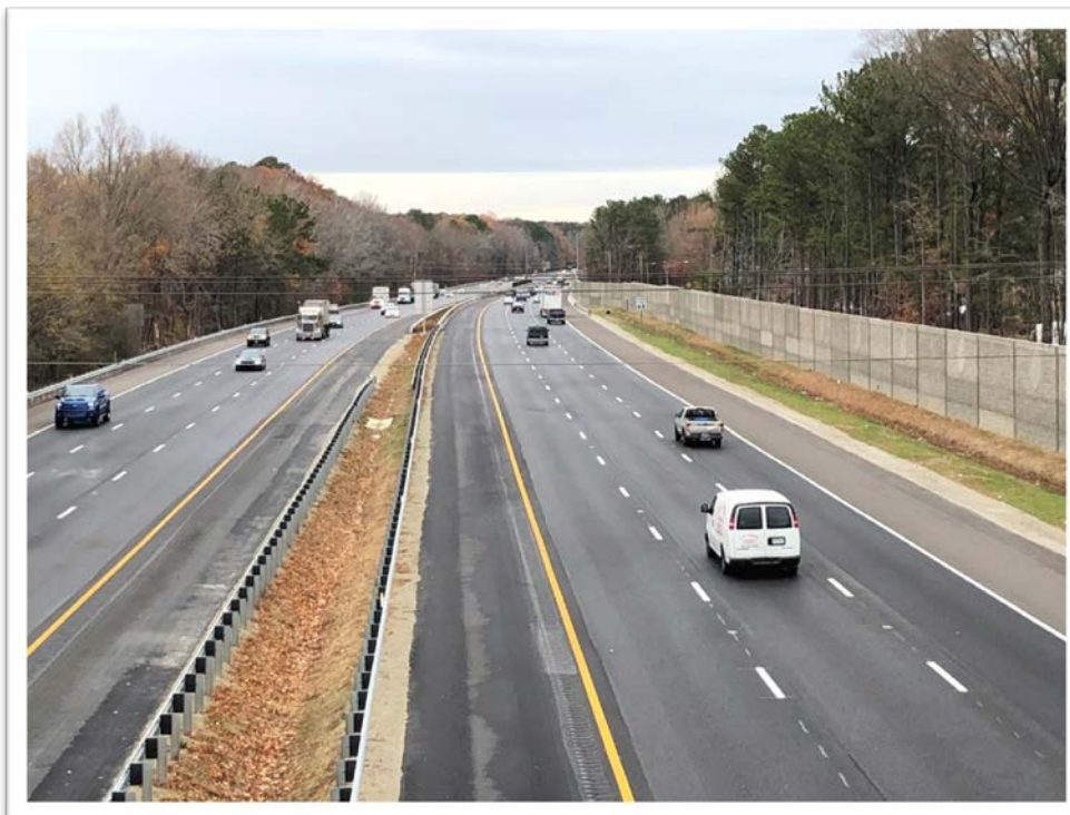
Project Site (Looking West from Denbigh Blvd.)
