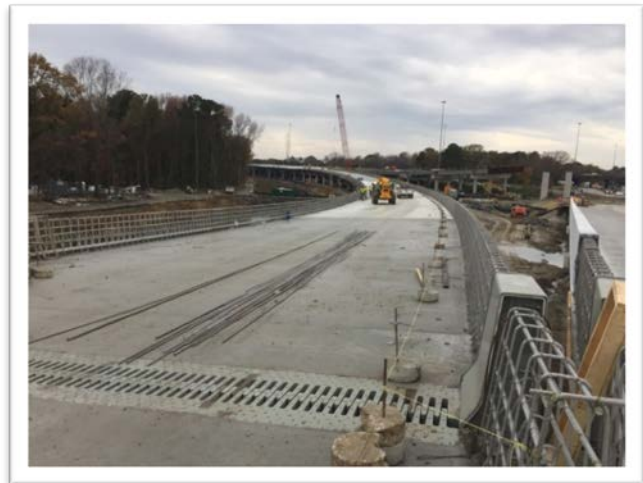
Recently completed Bridge B-603 deck sections
