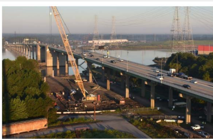
Pile Driving Operations for East Approach Spans of New High Rise Bridge
