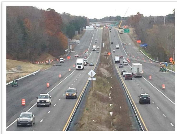
I-64 construction looking east from the Rt. 199 overpass
