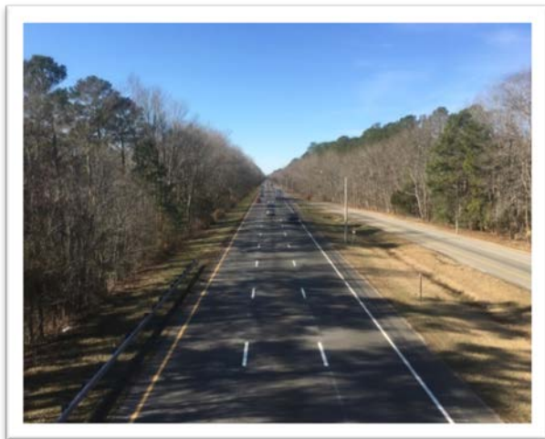
Existing facility looking westbound from weigh station
