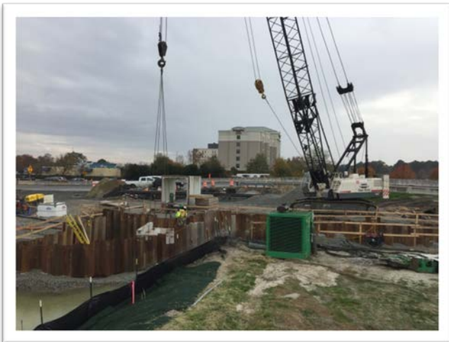
Setting last remaining sections of Culvert 8-34
