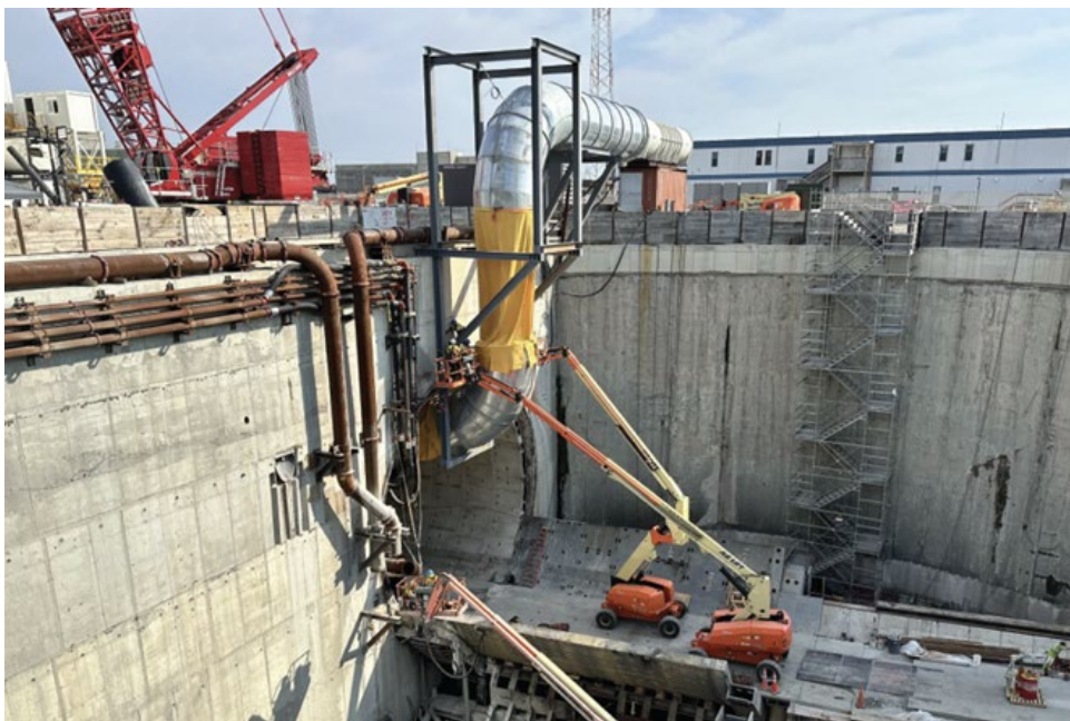
◀ HT Tunnel Steel rings and thrust frame removed during shaft reconfiguration
