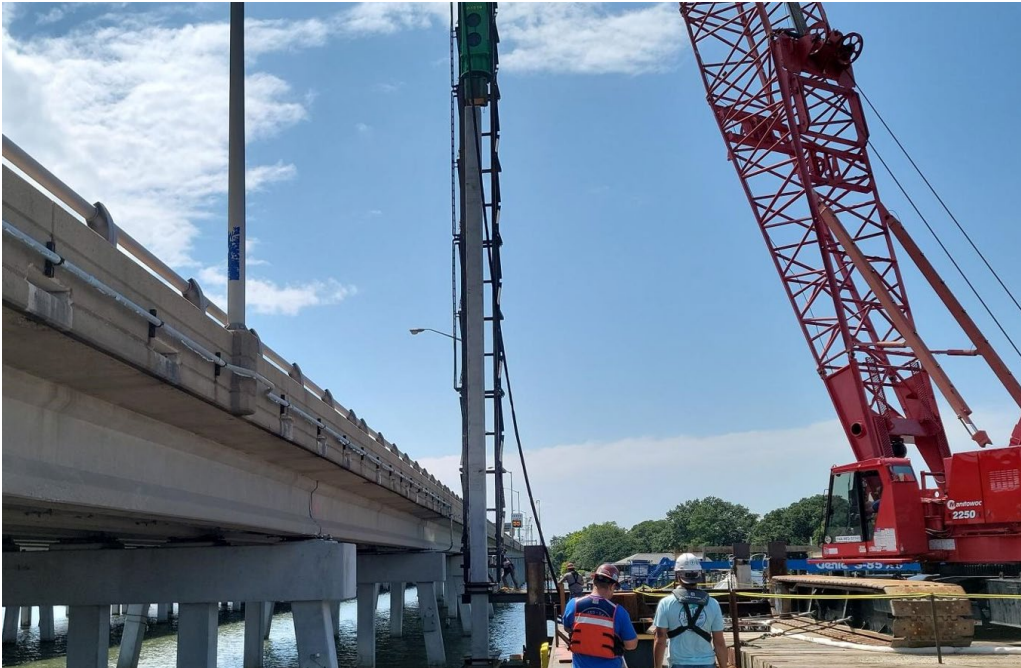
◀ Willoughby Bay Bridge Westbound Pile driving at Bent 16
